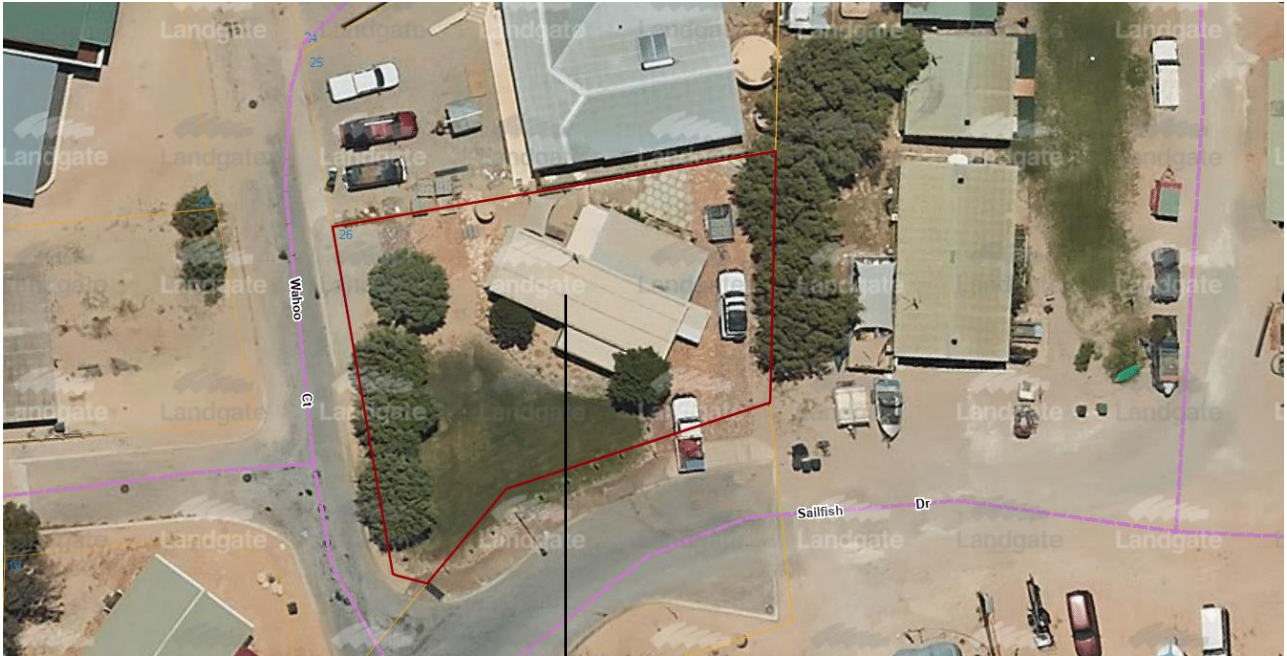
Figure 1. Lot 26 Sailfish Drive showing the dwelling to be demolished.
