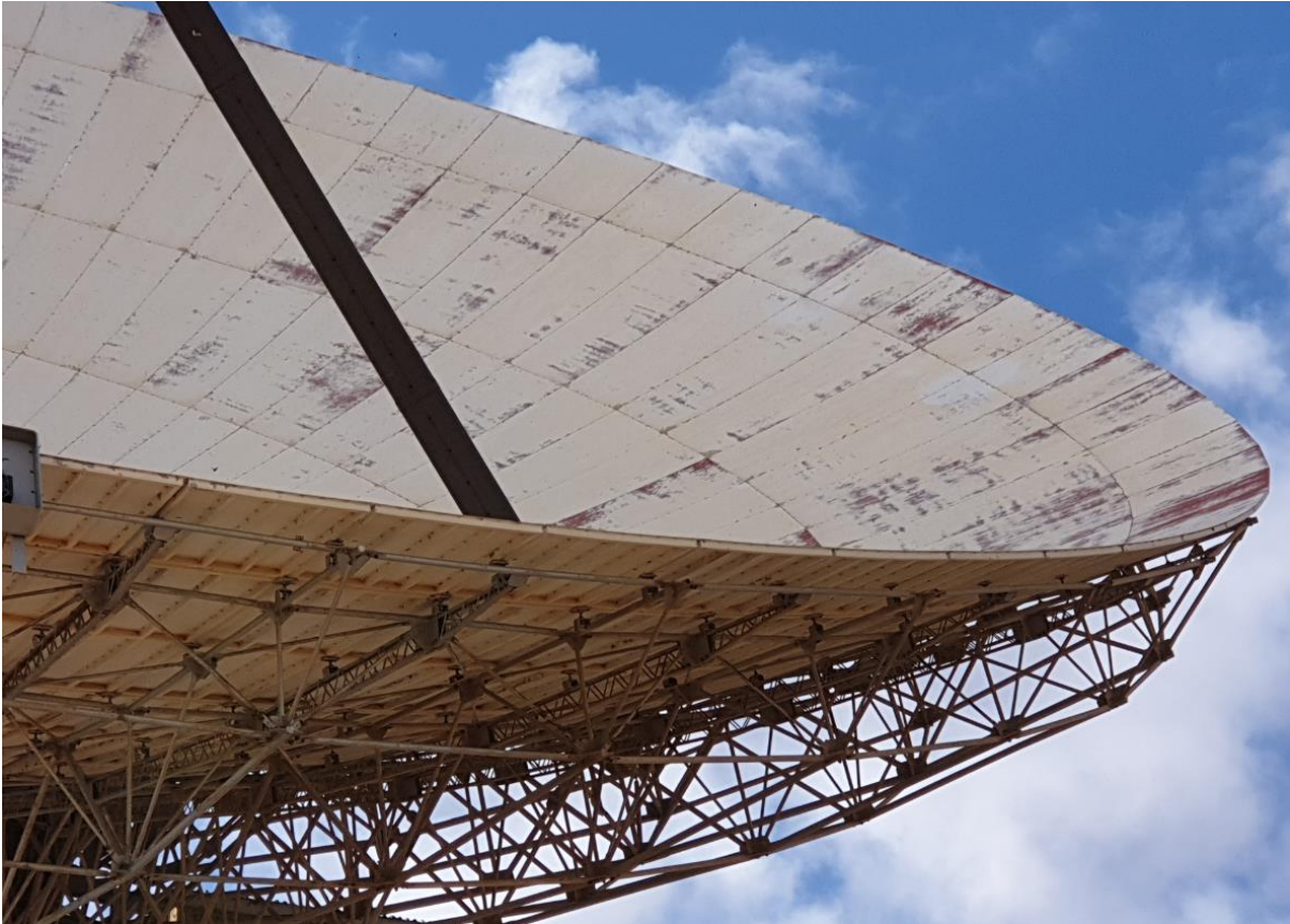
Figure 9: Dish reflector surface.
