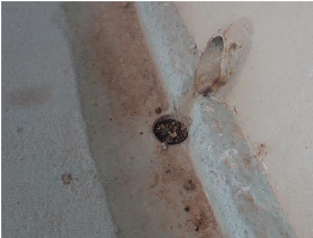
Figure 22: Blocked walkway drain.
