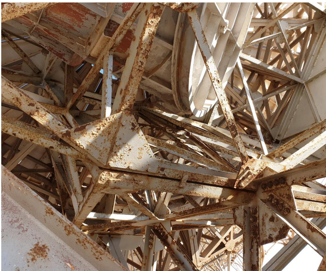
Figure 23: Vertical rotating assembly steelwork condition.
