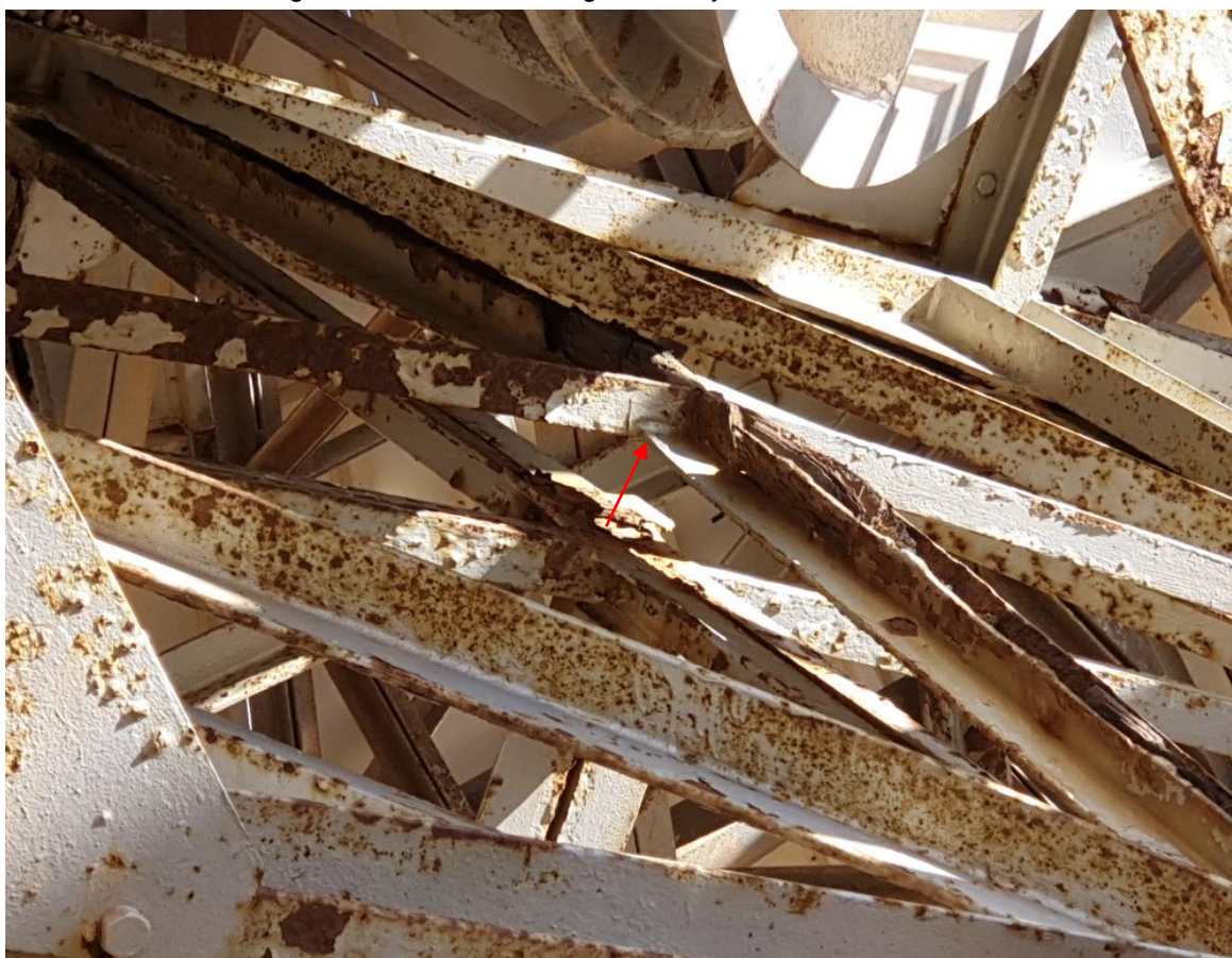
Figure 24: Vertical rotating assembly deteriorating steelwork.
