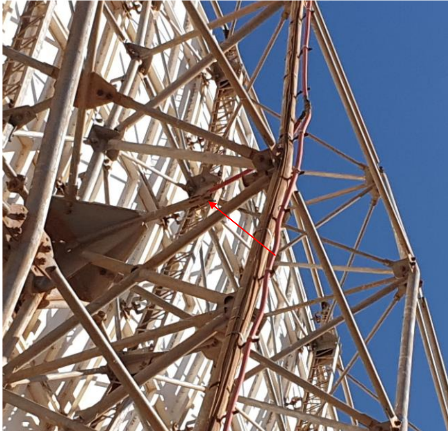
Figure 25: Space frame member failure.
