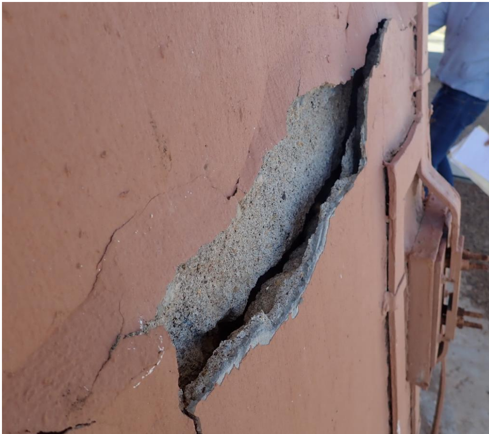
Figure 16: Concrete pedestal cracking and spalling concrete.
