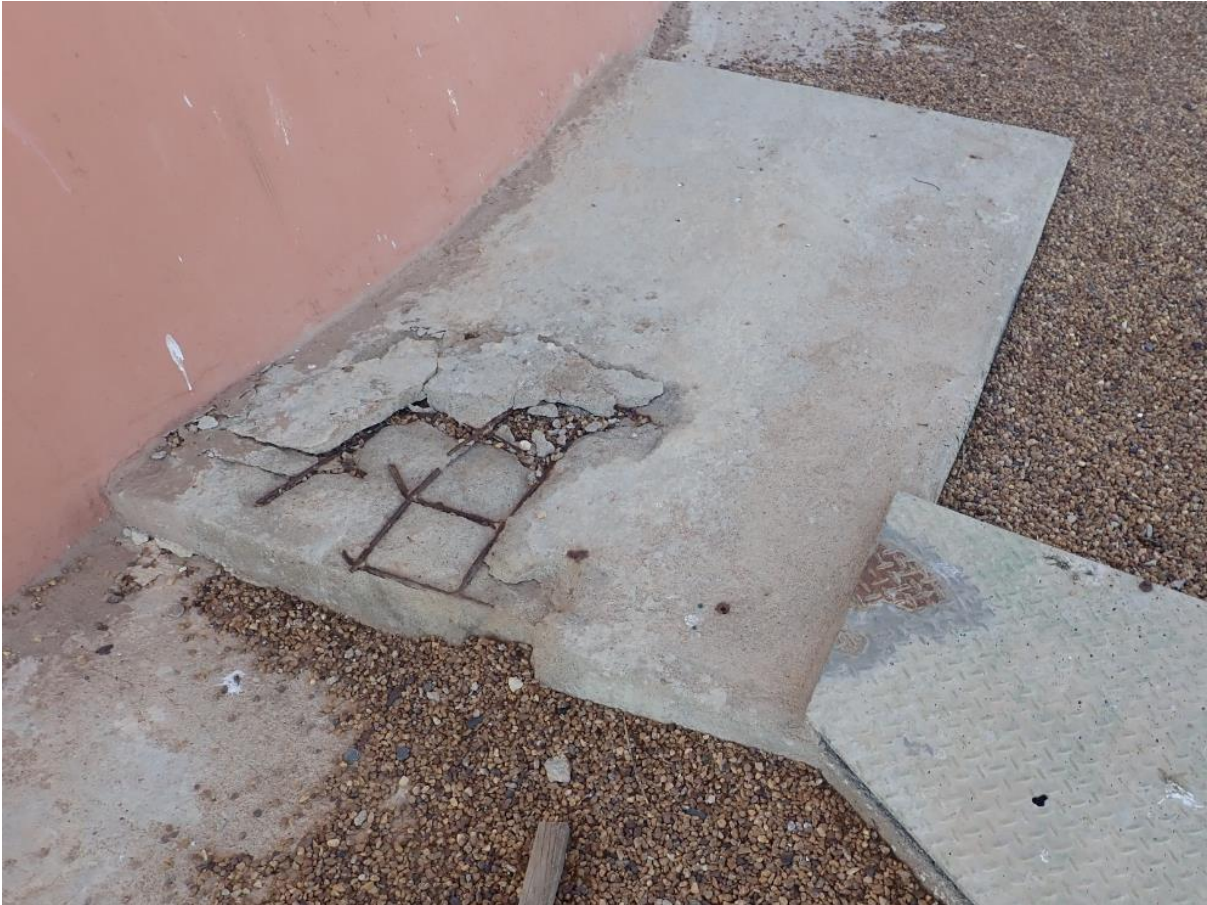
Figure 17: Repair cracked concrete on services lid at ground level.
