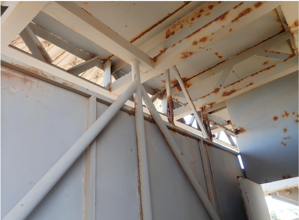
Figure 32: Hanging platform support frame.
