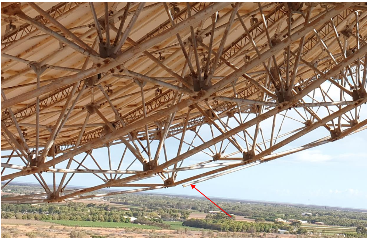
Figure 26: Space frame member failure.
