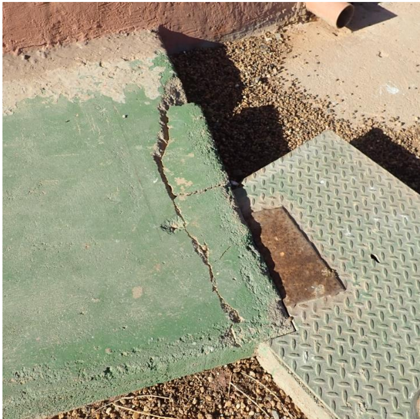
Figure 18: Repair cracked concrete on services lid at ground level.
