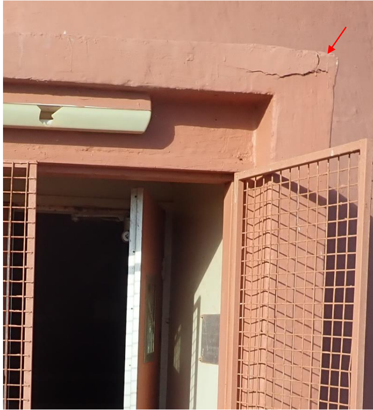
Figure 21: Access door opening top corner cracking.
