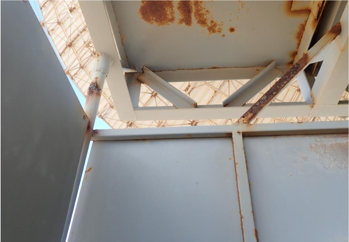
Figure 33: Hanging platform support frame.
