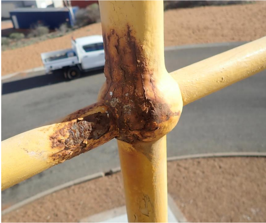
Figure 19: Pedestal walkway stanchion corrosion.
