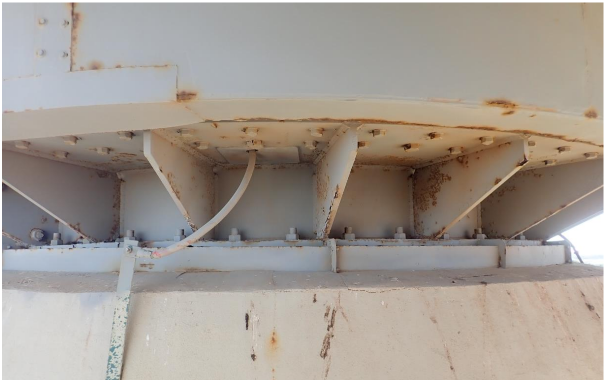
Figure 4: Azimuth rotating assembly.
