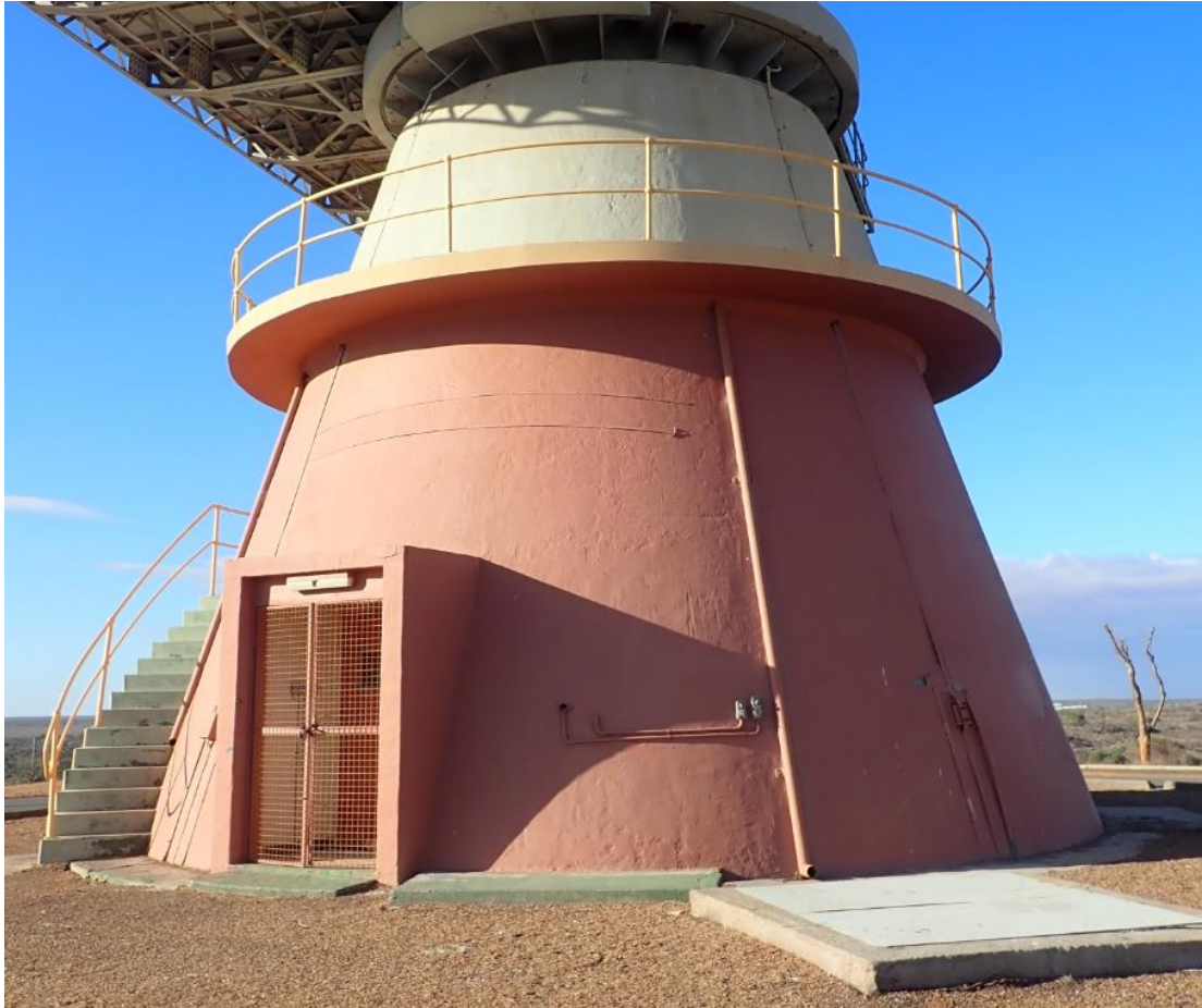
Figure 3: Concrete pedestal.
