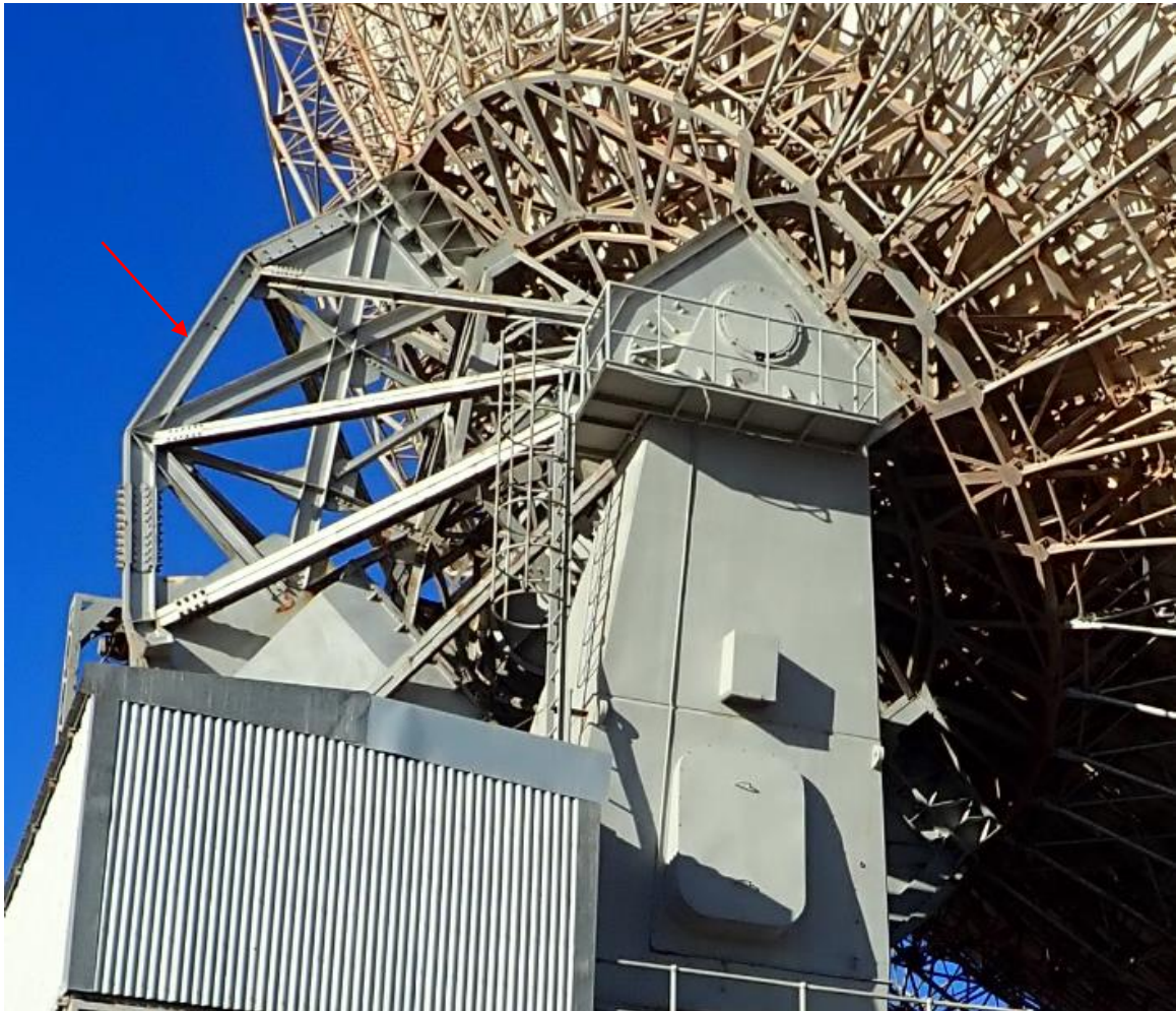
Figure 6: Vertical rotating assembly.
