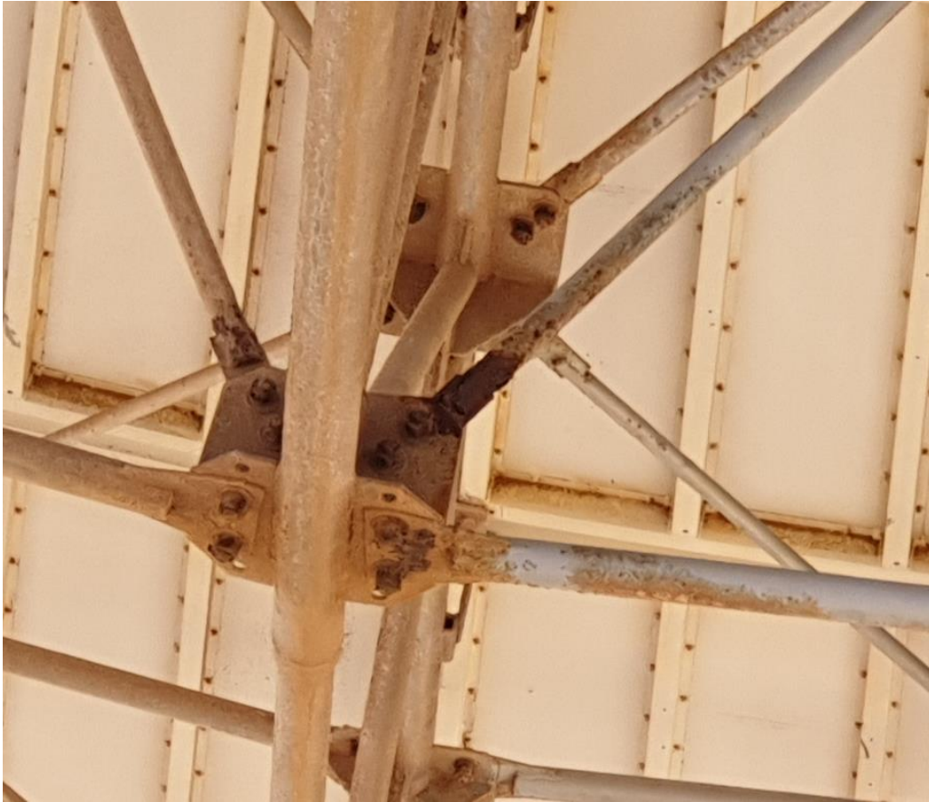
Figure 27: Space frame connection corrosion.
