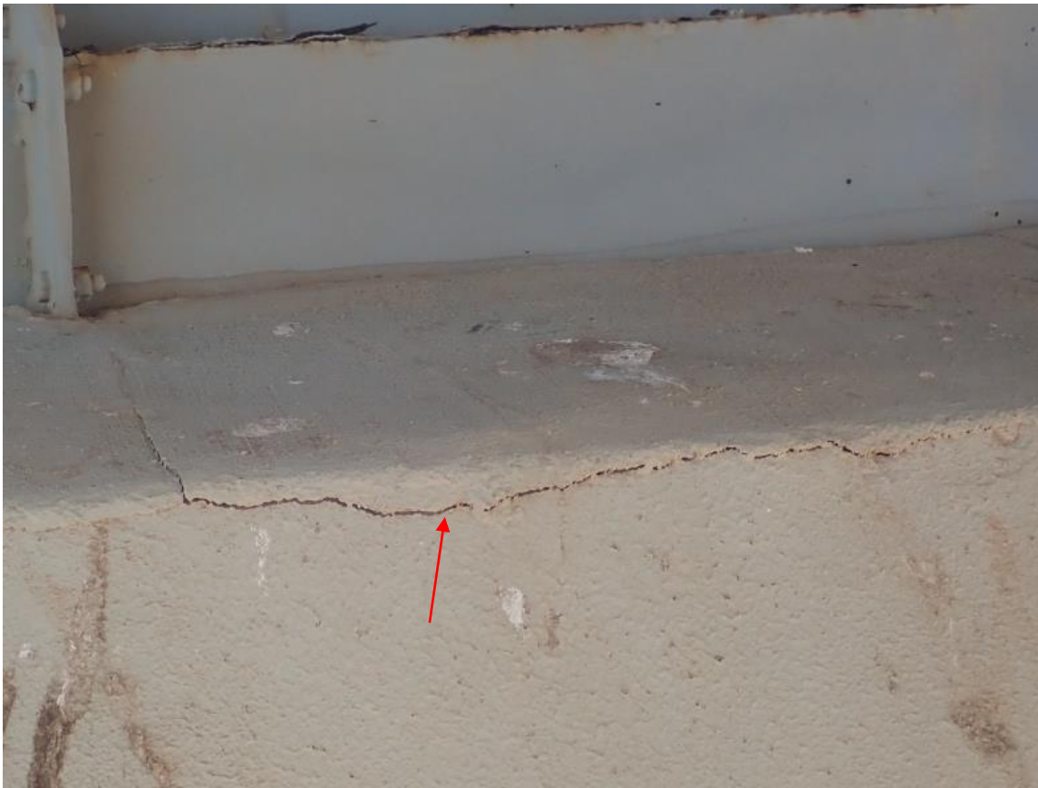
Figure 20: Pedestal top surface concrete cracking.
