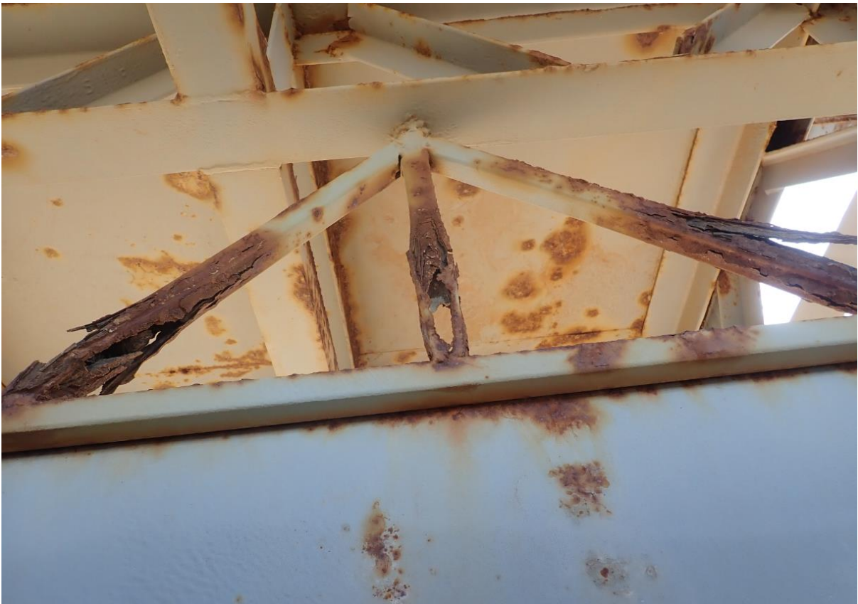
Figure 34: Hanging platform screen wall 25SHS frame corrosion.
