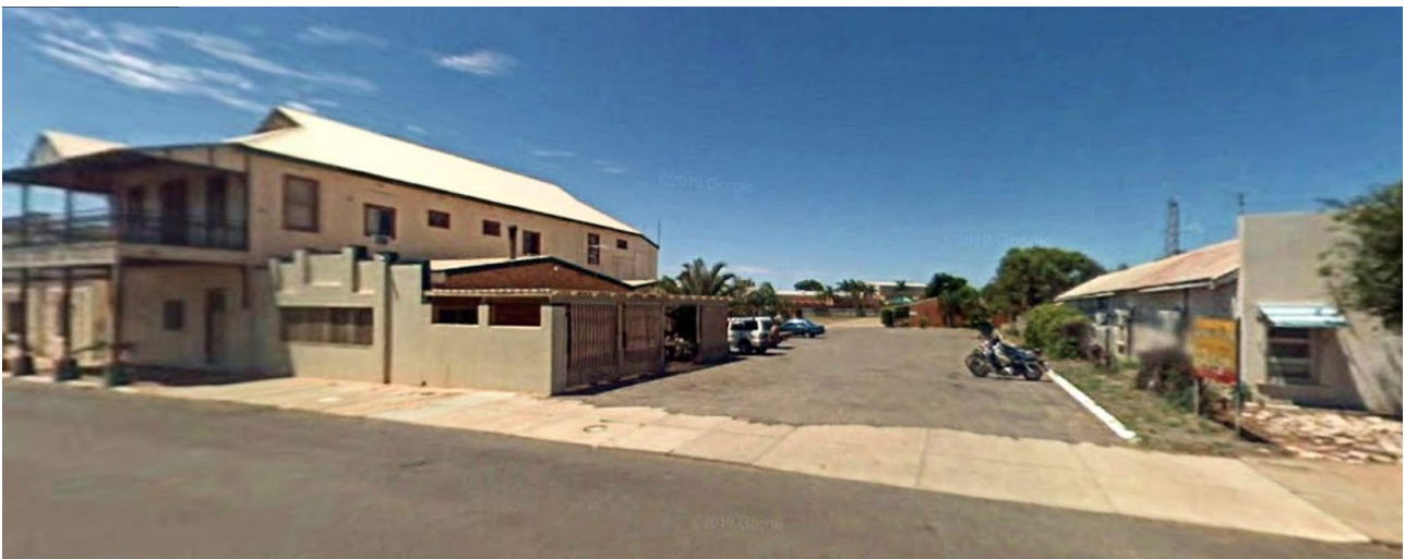
Figure 1: Olivia Terrace street frontage
