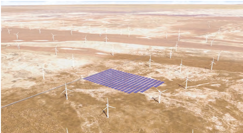
Figure 8. Renewable Energy Facilities
