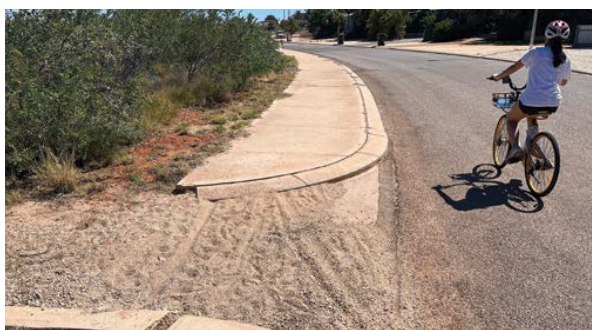
Drainage/spillway channels disrupting path continuity in Exmouth.
