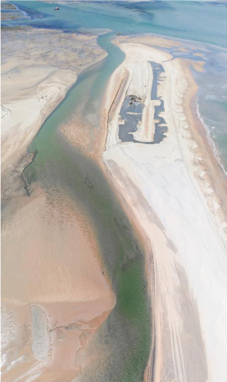
Spit stabilisation works.
