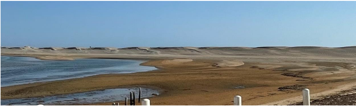
Newly constructed dune taking form.
