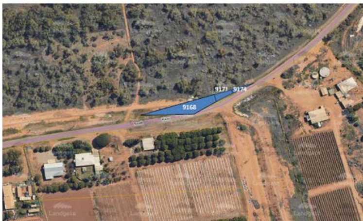
Road dedications – Adjacent No. 450 South River Rd., South Plantations
