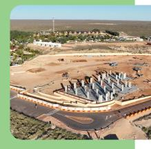
Recent milestones include the completion of concrete columns and ground slabs for the new Clubhouse and Reception building. Over the coming weeks, pre-cast beams and wall panels will be installed, while additional groundwork continues to prepare the site for the arrival of modular accommodation units later this year.
