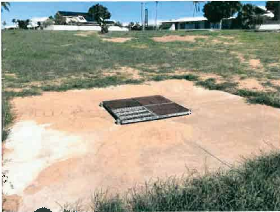
Photograph 5: Soakwell near the centre-west boundary of the site
