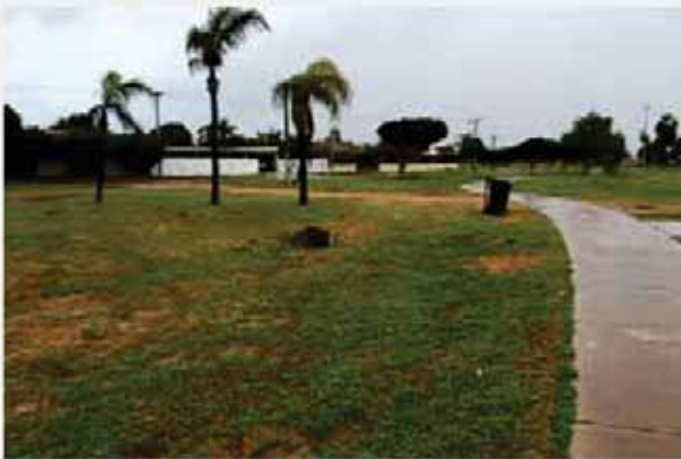
Existing drainage outlet within Structure Plan Area
