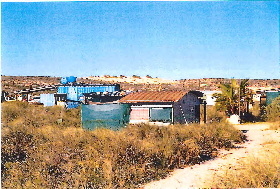
Figure 3: Vegetation Management- these shacks are not defensible in a fire situation
